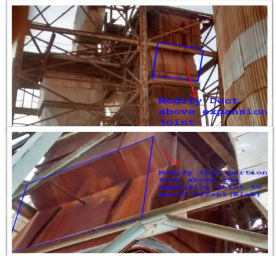
GCT to BH duct modification
